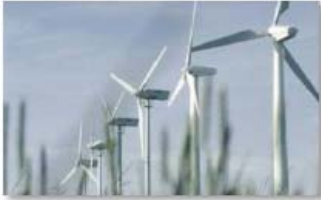
Connected Energy Management
